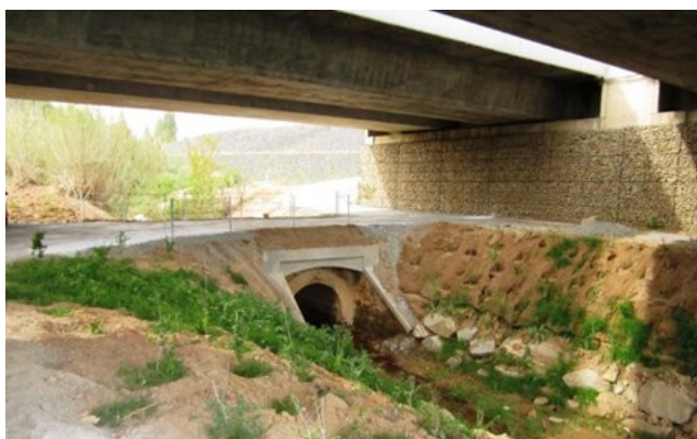
Close-up of the adaptations executed at the mixed structure built on road BP-1413 where it crosses the Torrent del Bosc and includes pedestrian crossings.
