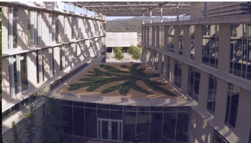
Green roof on the SENER corporate building in Parc de l'Alba.
