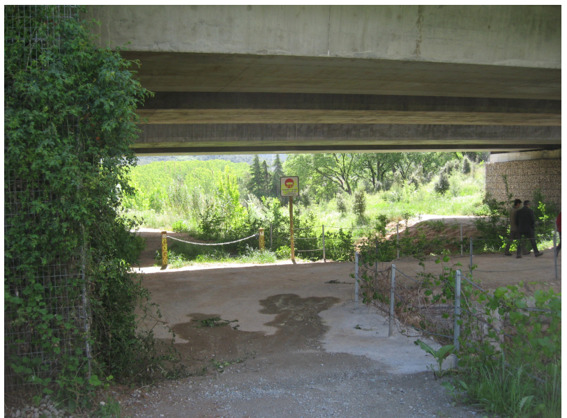
Passage of the Torrent de Bosc under road BP-1413. Mixed path for pedestrians, bicycles and fauna.
